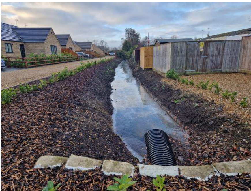
Photo showing retained water levels in ditch alongside Nos 30-38 Townley Close, rear of Nos 10-28 (26/01/23)
