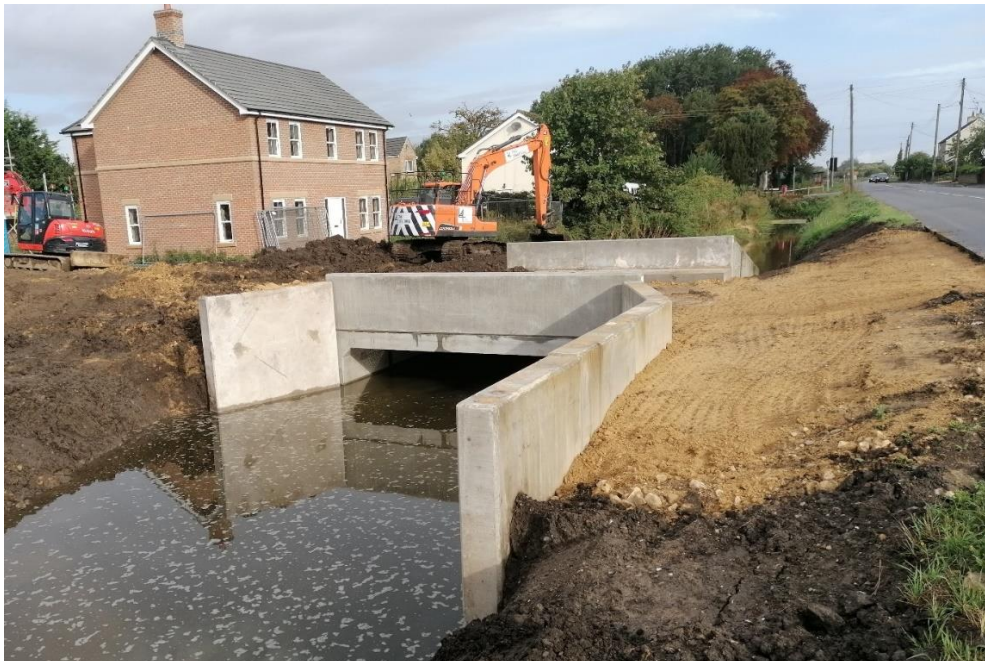
View of the access culvert viewed from the upstream end
