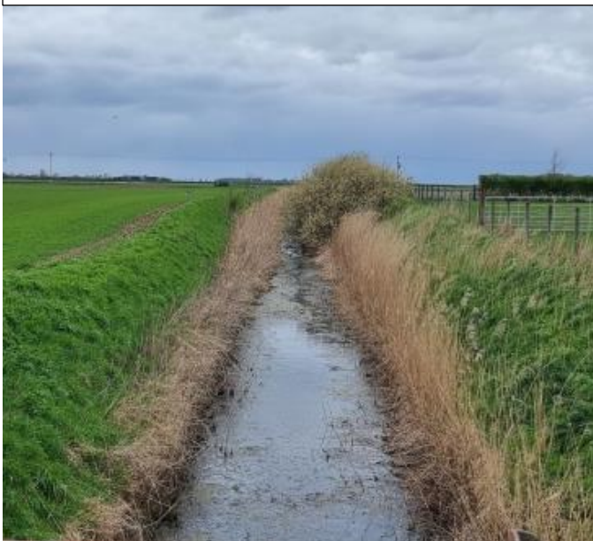
Point 16, Typical board drain in good order
