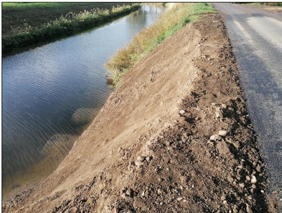
Completed Main Outfall Culverts Installation at Point 1 on Downstream Side
