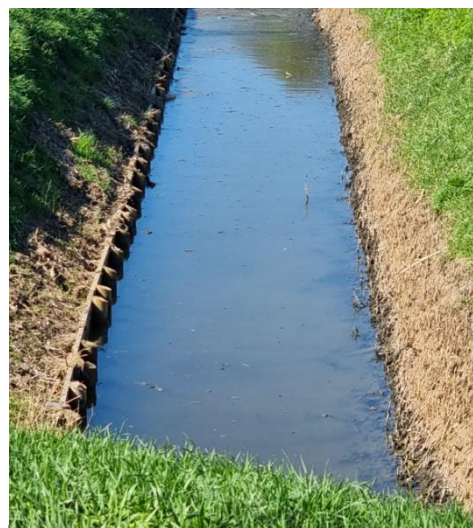
Revetment works, Point 38
