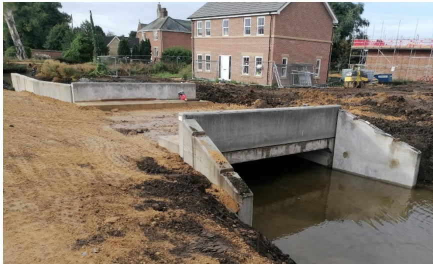
View of the access culvert viewed from the downstream end
