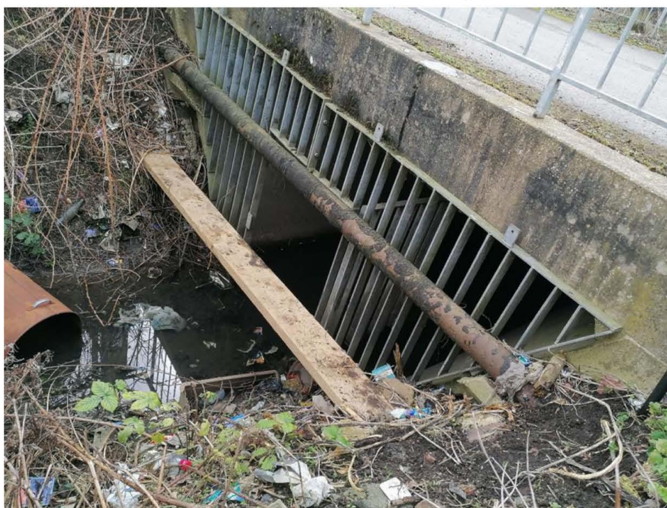
The access into Wisbech Business Park features a vertical screen and a duct crossing the channel Note the sloped concrete sides
