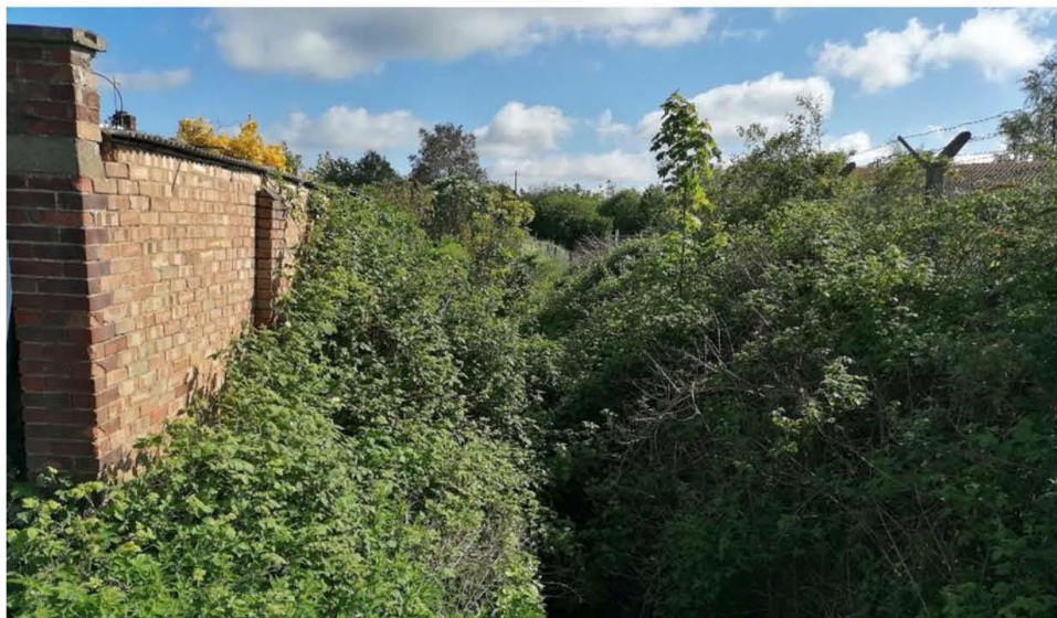
The Board's Drain viewed from the access into Wisbech Business Park looking upstream toward Hillburn Road
