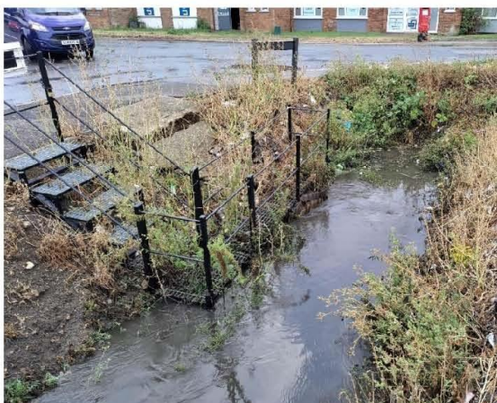
Halfpenny Lane Drain viewed from New Drove (Point 55)
