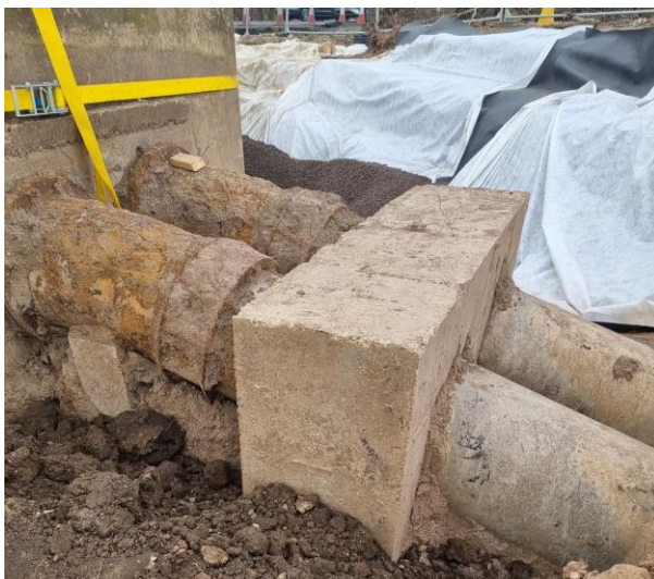
Views of the exposed rising main as it enters the surge chamber
