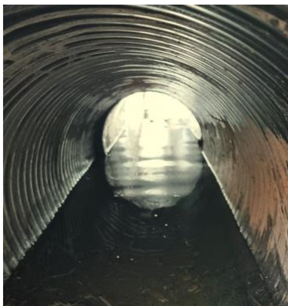
New twin wall plastic liner
