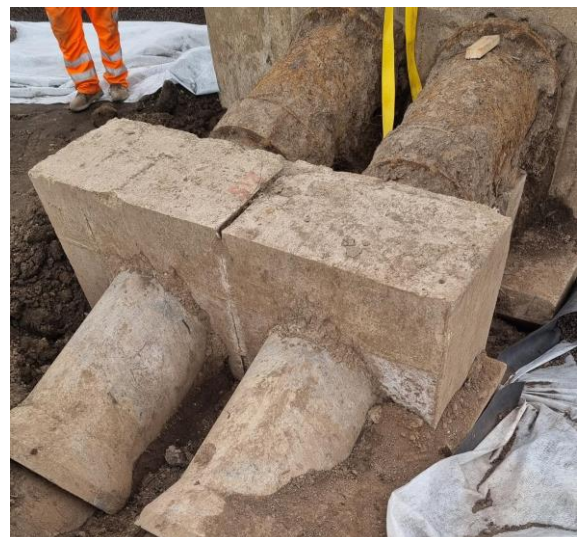
Views of the exposed rising main as it enters the surge chamber
