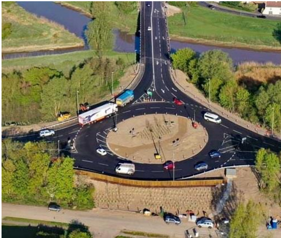
Extract from National Highways Press Release photograph showing the completed works. The Rings End Pumping Station Surge Chamber is visible toward the bottom left hand corner.
