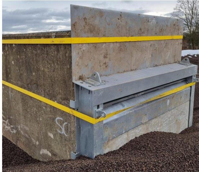
A view of the fabricated steelwork protection structure strapped to the surge chamber during backfilling to form the eastern embankment of the roundabout
