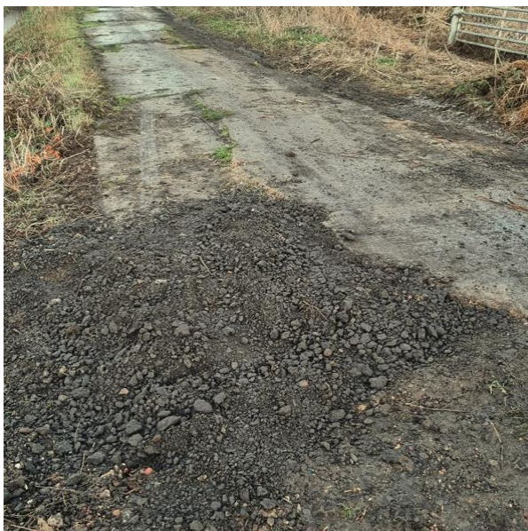
Remedial repairs to public byway
