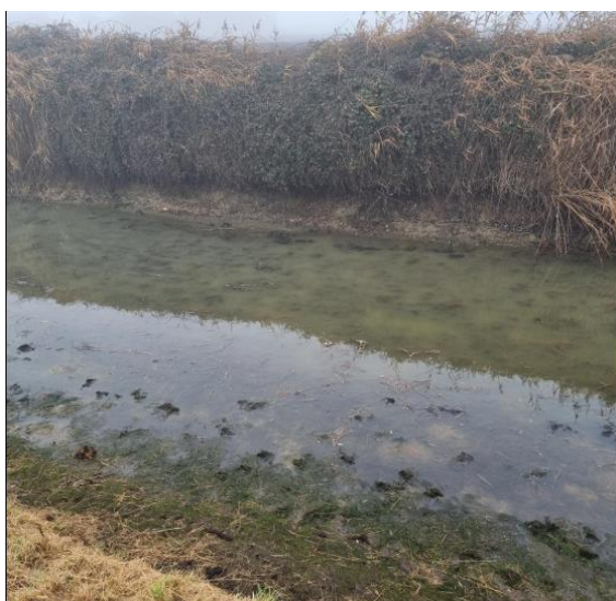
Large accumulations of silt and aquatic weed, exposed during the winter pump down for machine cleansing works on Ash Drain
