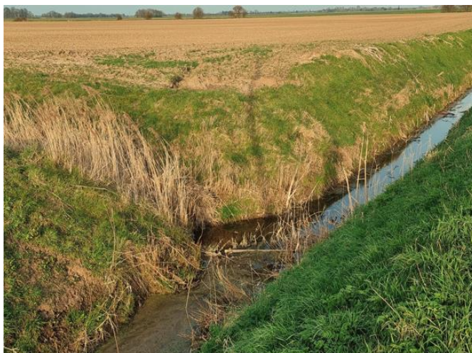
Inlet culvert, reach 10-11
