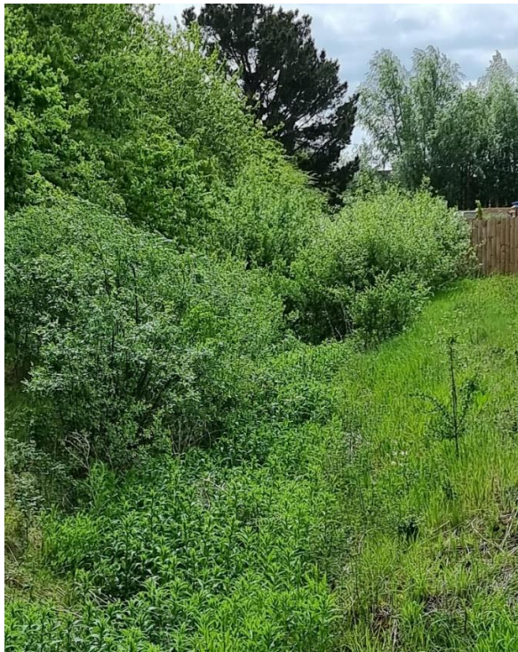
Current view of the upstream end of Bridge Lane Drain
