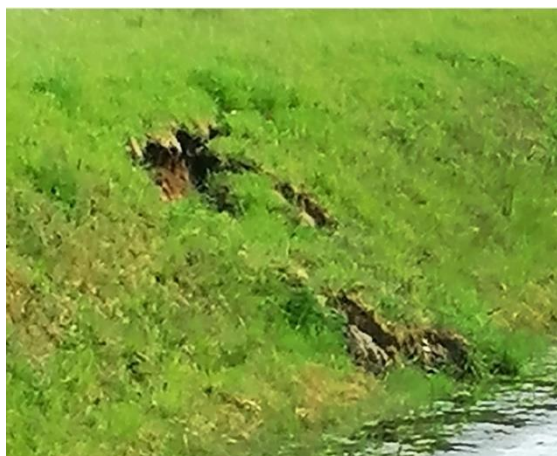
2021 EEDA Drain, reach 19-20
