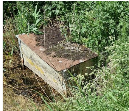
Division Dam @ Point 10
