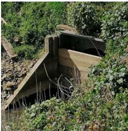
Division Dam at Point 69
