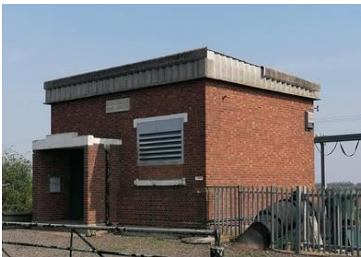
Damaged Asbestos Roofing at the Pumping Station
