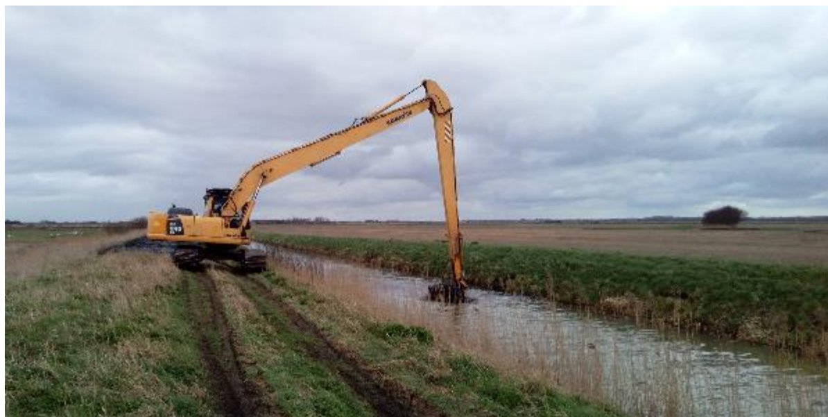
Maintenance Dredging New Dyke – February 2020
