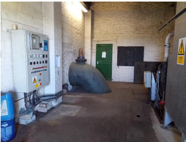
Control panel diesel engine/pump
