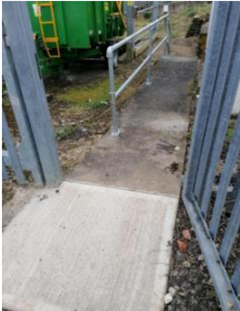
Replacement slab in gateway and new hand rail at Pumping Station
