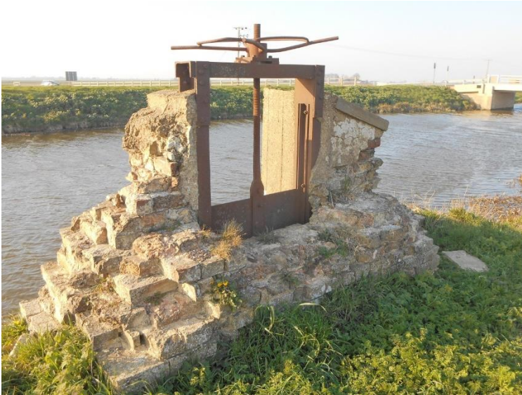
View of headwall and penstock on upstream/ riverside end of arch
