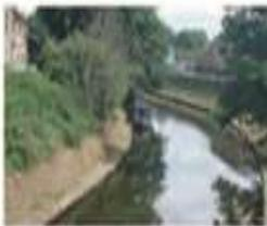
Because boat wash is a major cause of bank erosion - the faster a boat goes, the greater its wash and the faster the banks will erode. The Middle Level area depends, for its flood protection, on artificial flood banks and any erosion of these banks greatly increases the risk of the land and properties flooding. Also, the silt washed from the banks has to be expensively dredged from the waterways in order to maintain sufficient depths for the boats to continue to navigate the waterways.
