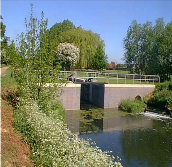
Boats in the lock must be held at least 1.0m (3'-3") clear of the upstream doors to avoid fouling the sill as the water level is lowered and well away from the downstream doors to avoid entrapment beneath the penstock/paddle/slackers access walkway when the water level is raised.
