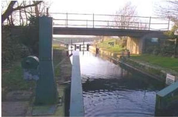
Ensure that the lock doors and penstocks/paddles/slackers are properly closed after use. Leakage can rapidly lower the water level in Well Creek, which can sometimes require several days to restore a satisfactory navigation level. To assist in maintaining adequate water in the Creek, 'double-up' where possible when negotiating the lock.
