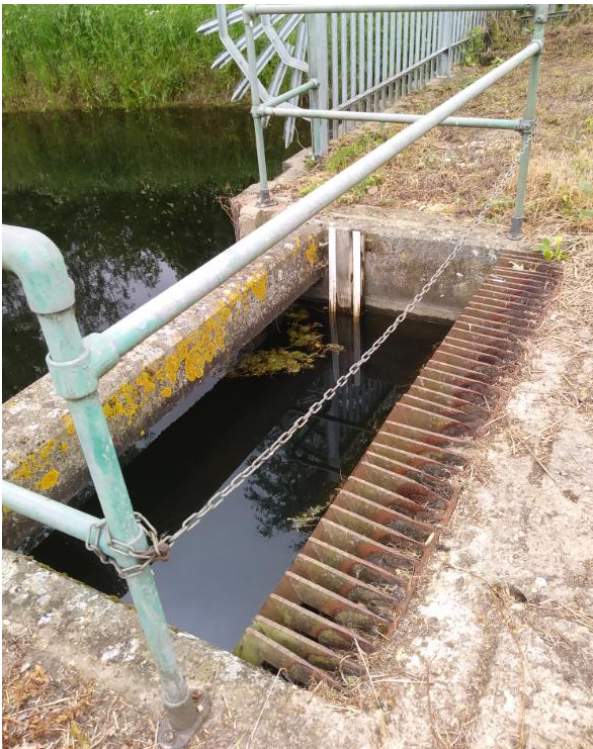
Handrail improvements at Norwood pumping Station
