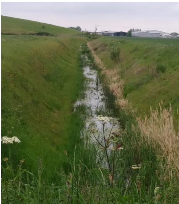
EEDA Drain, reach 19-20
