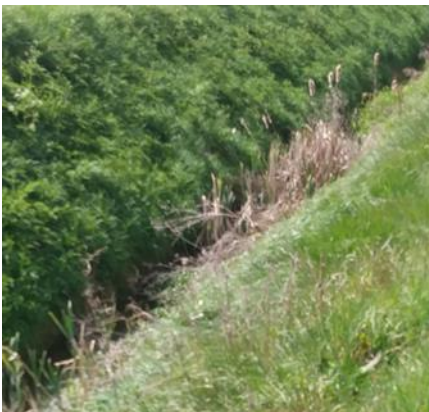
Reeds & Emergent weeds, requiring an application of Roundup herbicide
