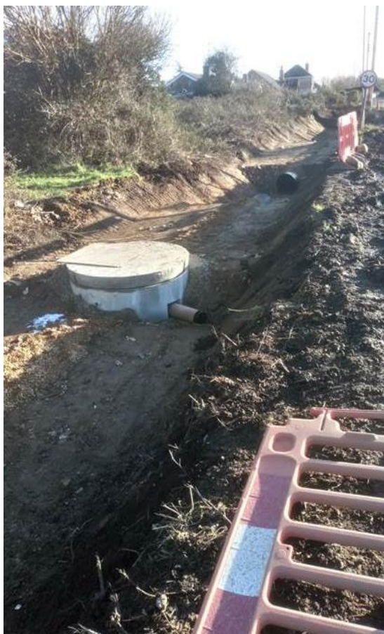
One of several photographs of the works supplied by the complainant
