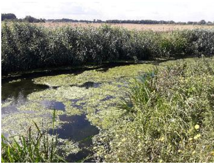
Pig Water Drain – machine cleansing was required to remove filamentous algae, (cott) from the water channel on three separate occasions during the summer. The entire length of the watercourse required machine cleansing on the third round, to remove dense infestations from the upper reaches between Horsey Toll Sluice and Farcet Overspill. The channel forms a vital link for summer water transfer for subsequent abstraction in the Bevills Leam pond.
