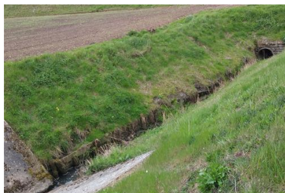
Bank Subsidence, reach 36-37
