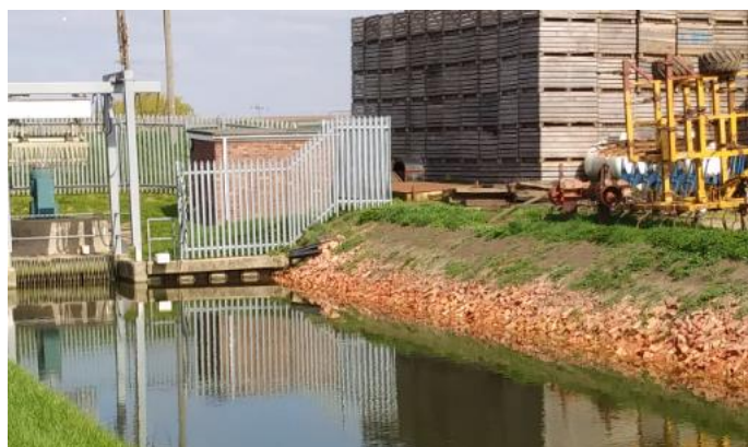
Beggars Bridge Pumping Station Revetment works
