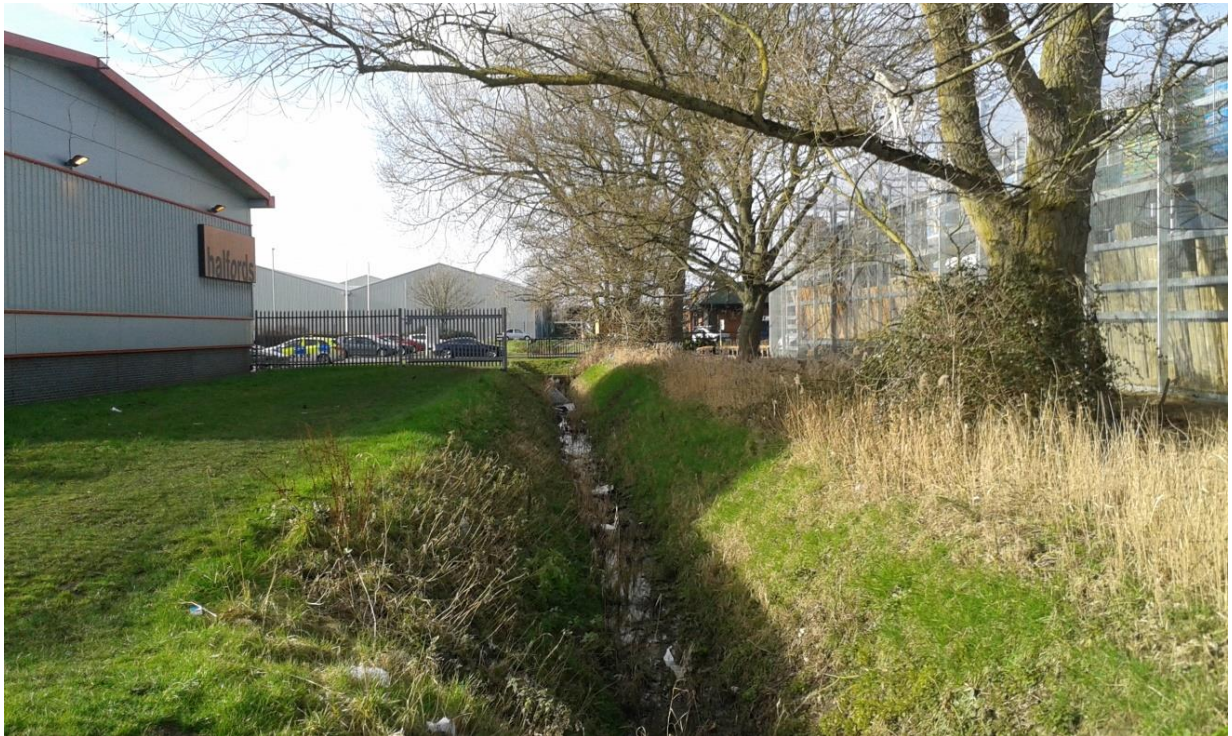
View of the Board's Drain looking toward Cromwell Road showing the existing maintenance access strip beside Halfords
