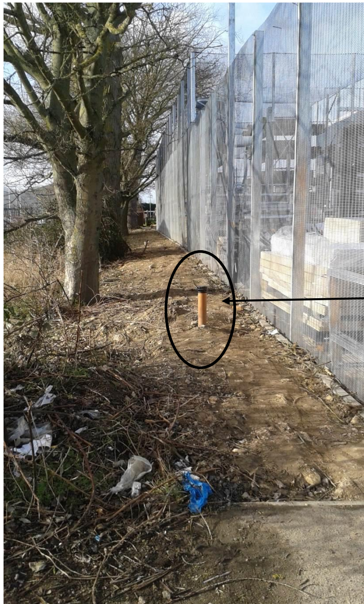
View of the breather pipe for the buried attenuation tank
