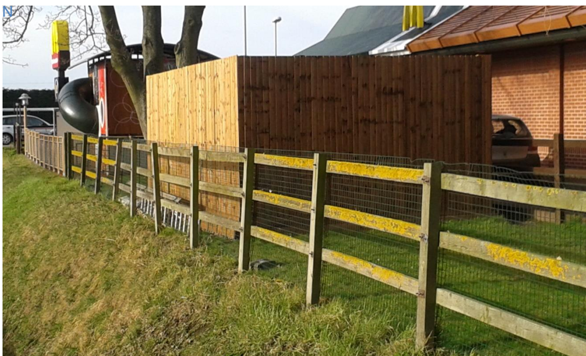
Photograph of the completed works within the maintenance access strip
