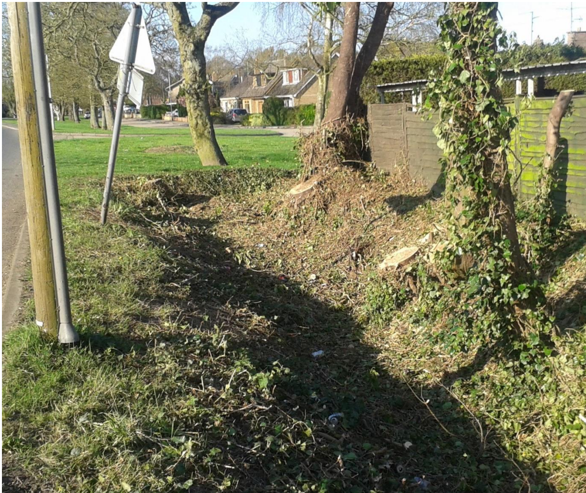
Photograph of the upstream end of the private roadside watercourse beside Fridaybridge Road following the removal/reduction of trees and other vegetation
