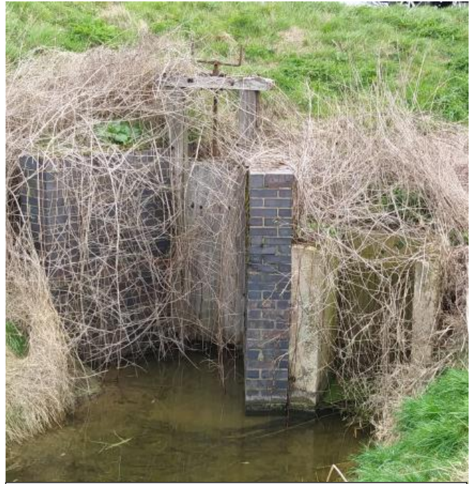
Gravity outfall at Point 35
