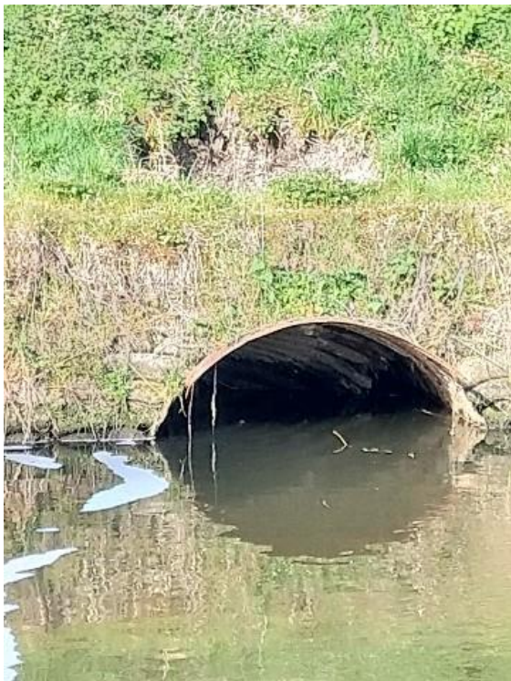
Two views of the collapsed section of the outfall prior to mitigation being undertaken
