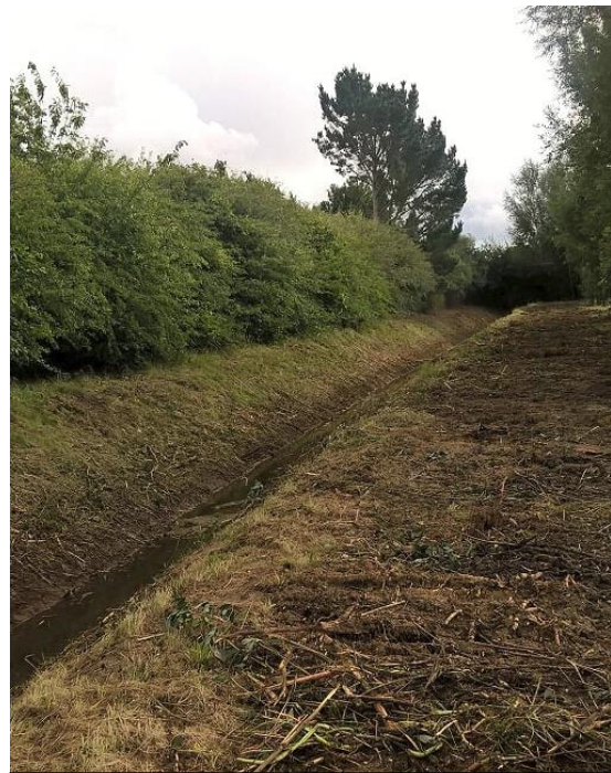
Reach 80-81 following the cutting with a forestry flail & machine cleansing works
