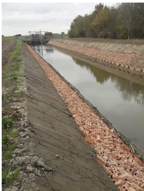
Duncombes Main Pump Drain
