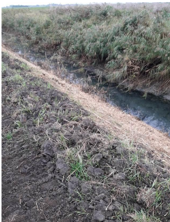
Damage to the top of the bank, hindering flail mowing works and threatening the bank's stability
