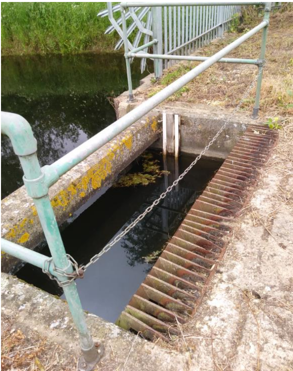
Handrail improvements at Norwood pumping Station
