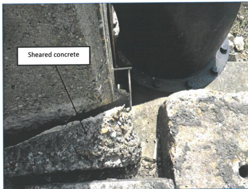
13. Detailed view of the sheared nib and fresh face of concrete.
