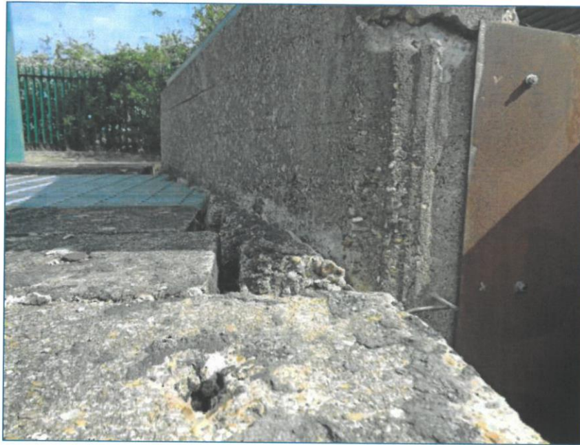
11. Shows the area of sheared concrete.
