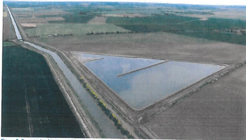
Figure 3: Dewatering lagoon at the 40ft drain project, Boston (Swineshead), UK
