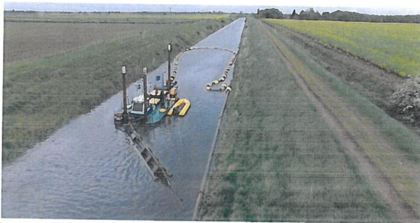
Figure 2: 10' Cutter Suction Dredger at the 40ft drain project, Boston (Swineshead), UK
