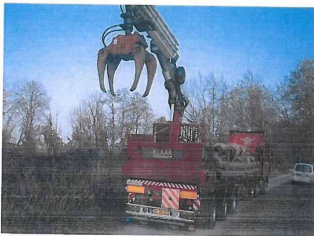
Figure 5: Special pipe trailer used for installation of the pipelines
