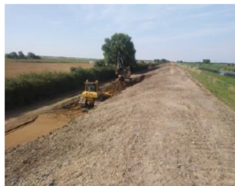
Cutting a bench layer on the SLBB at Sutton Gault
