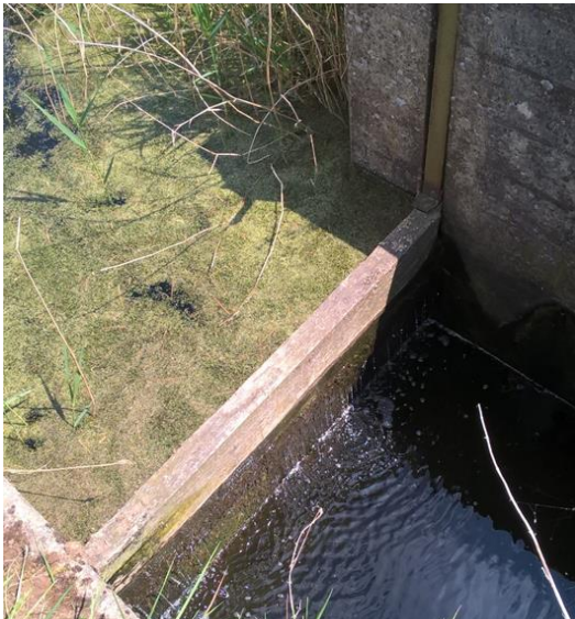
Water Control Structure Point 75
