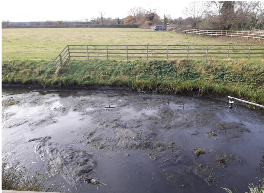
Cott build up at Pump Basin prior to machine cleansing
