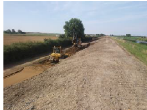
Cutting a bench layer on the SLBB at Sutton Gault
