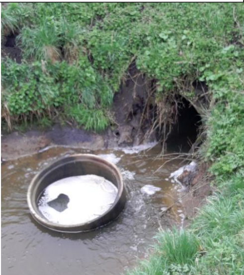
Dislodged Concrete Culvert pipe Reach 15-18
