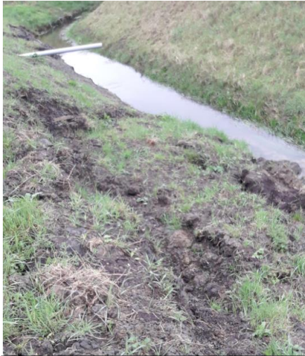
Campole Drain Subsidence, Reach 22-23
