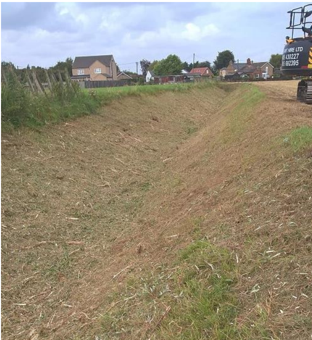
Lilyholt drain, reach 92-94 after the sapling removal
