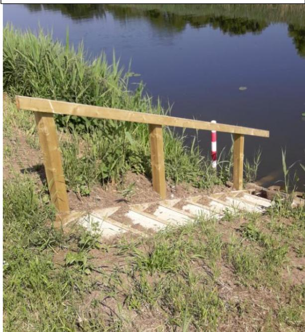
Following the Chairman's prior approval, a set of concrete steps has been installed at the Commissioners' gravity outfall at Point 13. The steps are required to improve pedestrian access to the structure and ensure the Commissioners are compliant with current Health & Safety guidelines. The outfall flap valve has also been repaired.
