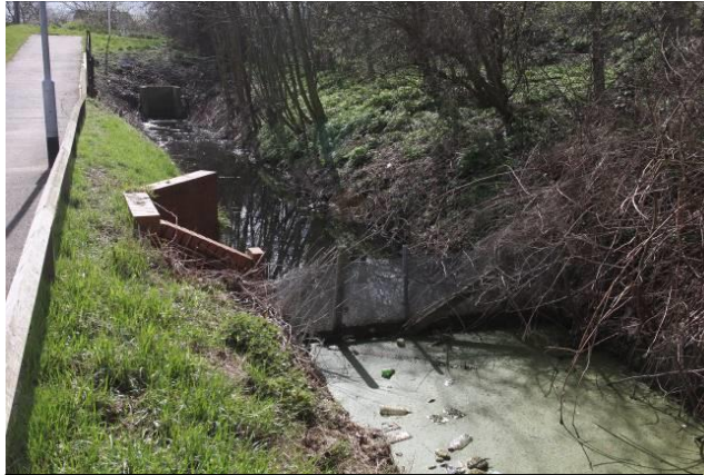
Above, the mesh screen at point 13 stops the spread of the invasive non-native plants in drain 4-5-6 while they are being controlled. This culvert at point 4 at Foxglove Way will require a similar mesh guard to prevent spread of the invasive plants towards South Creek Pumping Station drains, below.
