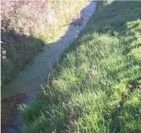
Bank movement on Reach 5-6
