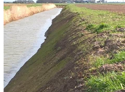
Bank Trimming Reach 9-10
