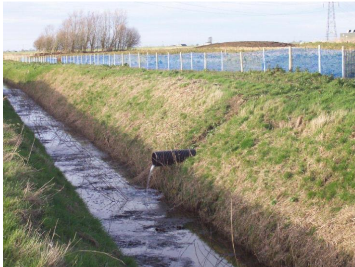
A view of the illegal fence and outfall pipe
