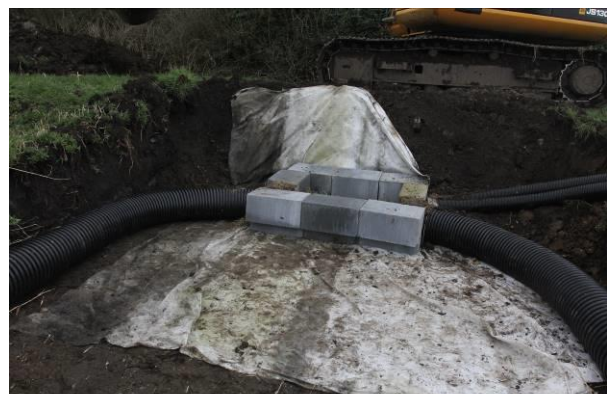
This was the 81st otter holt constructed as part of the Middle Level Otter Recovery Project.
