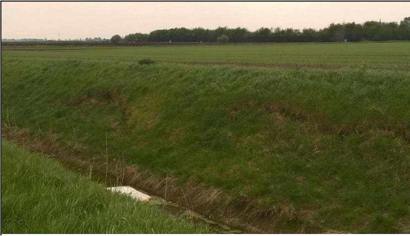
Bank Subsidence, reach 42-54
