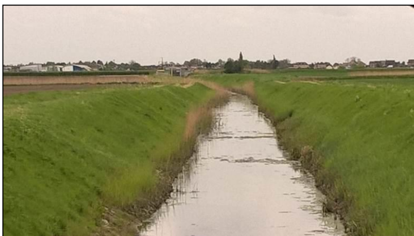
Curf Pump Drain, reach 80-81
