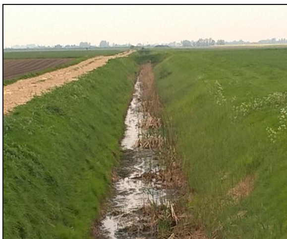
Normoor Drain, reach 73-74
