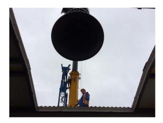
The general condition of the pump, which was some 33 years old and has operated some 23000 hours, was good and therefore as a consequence it was recommended that removal and inspection of any of the other pumpset (which have operated for considerably less hours), will not be necessary for a further five years.
