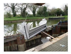
Ashline Lock - bypass weir works - following approval from the Executive Committee to proceed with the replacement of the existing gates an order was placed with HC Water Control for two stainless steel beamless drop down weir tilting gates. The new tilting gates were delivered on time by HC Water Control (at the end of March 2016) and installed using MLC labour during the first week in April. The performance of the gates to date has been very good.
