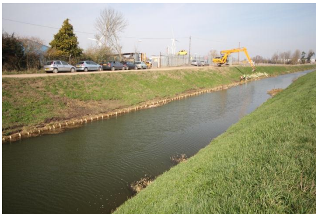
Coir roll installed as improved water vole habitat at Ramsey Highlode.
