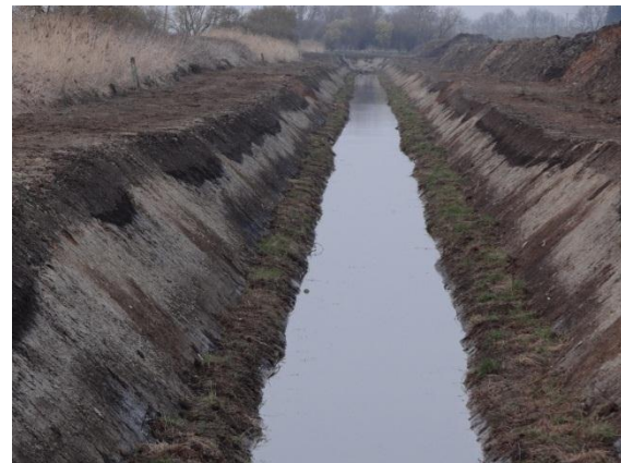
A new ditch with shelves designed to develop into replacement water vole habitat at Colne Fen.
