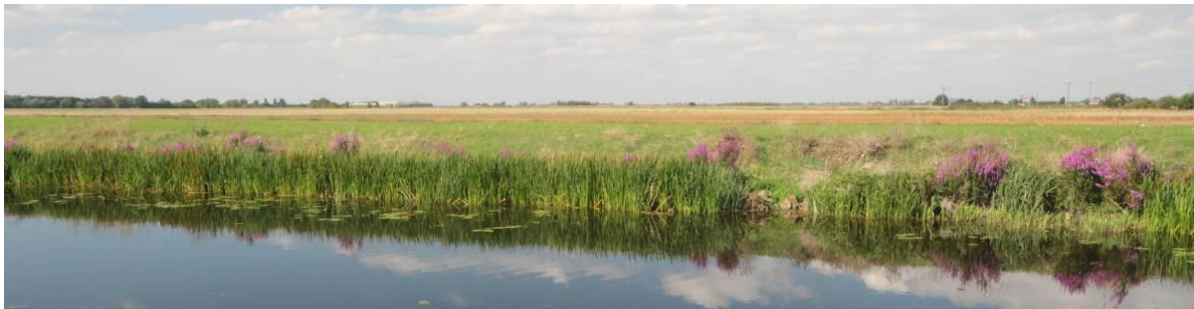
Coir rolls that were installed on the Sixteen Foot Drain at Bedlam Bridge in January 2005 continue to thrive and to provide good bank protection opposite the outfall from Bedlam Bridge Pumping Station.
