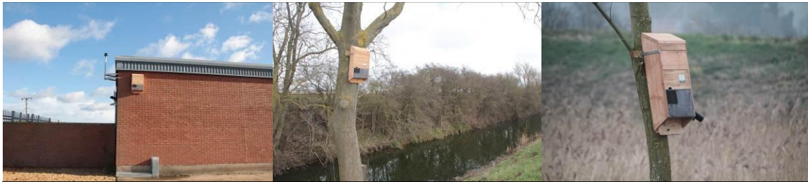
Above, bat boxes installed at Tebbit's Bridge PS, the Forty Foot near Horseway Locks & the reedbed at St Germans PS.
