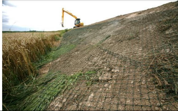
Left, the whole bank was rebuilt as badger holes had extended across it. Right, link mesh is pegged down prior to being covered with a thin layer of soil to prevent returns.
