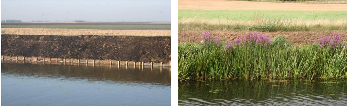
Coir rolls near Bedlam Bridge on the Sixteen Foot River, left, shortly after installation in 2009 and right, August 2011. Bur-reed has established naturally in front of the sedges, rushes and purple loosestrife that are growing out of the coir.
