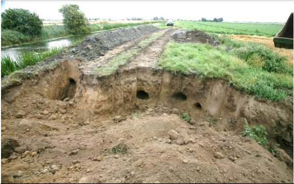
Left, the whole bank was rebuilt as badger holes had extended across it. Right, link mesh is pegged down prior to being covered with a thin layer of soil to prevent returns.
