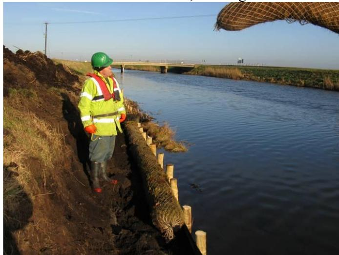
*Pre-planted coir roll revetment being installed near Bedlam Bridge.*
