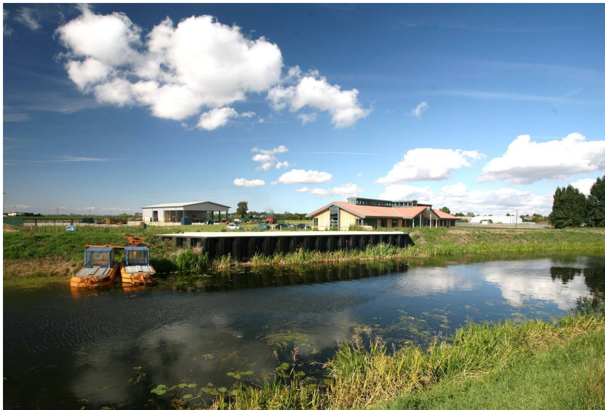
The new MLC Offices and depot.
