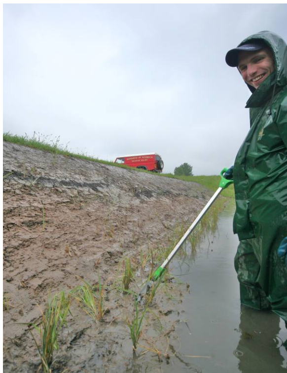
A wet job on a wet day. Ben Wales at Hundred of Wisbech IDB installs sedge plugs at a new ditch margin ledge to trial the method for the benefit of bank stability and biodiversity.
